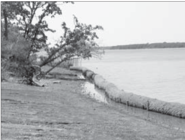
Coir roll breakwaters are held in place by wooden stakes.
