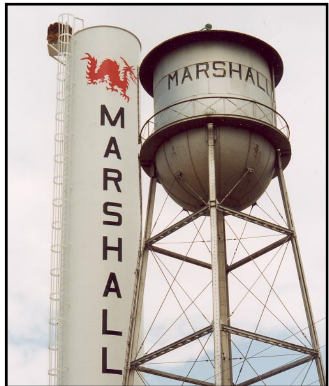
The OWRB's loan and grant programs were responsible for 75 percent of all state water and wastewater infrastructure financing in 2000. The Town of Marshall's new water tower (shown here in stark contrast to the old structure) was enabled through a $92,965 OWRB REAP grant as well as local funds contributed by both Marshall and the Association of Central Oklahoma Governments (ACOG).
