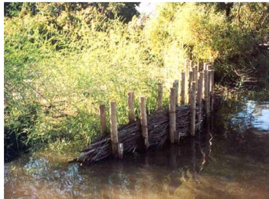
**Figure 2.18: Branchbox breakwater with vegetation behind, September 2001.**
