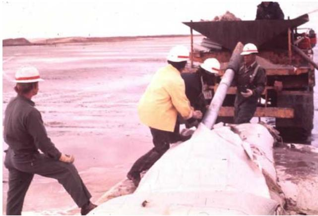
Figure 2.66: Geobags being filled to form a breakwater for planting wetlands behind it.
