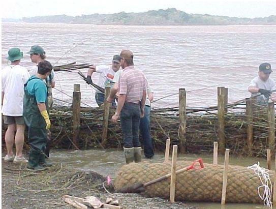
**Figure 2.17: Branchbox breakwater being constructed in April 2000.**
