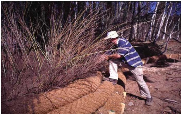
**Figure 2.13: CGRs and willow used to restore bank in figure above (Allen 2001b).**
