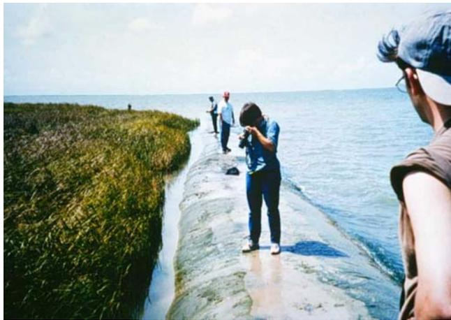
Figure 2.24: Geotube breakwater with planted wetlands.
