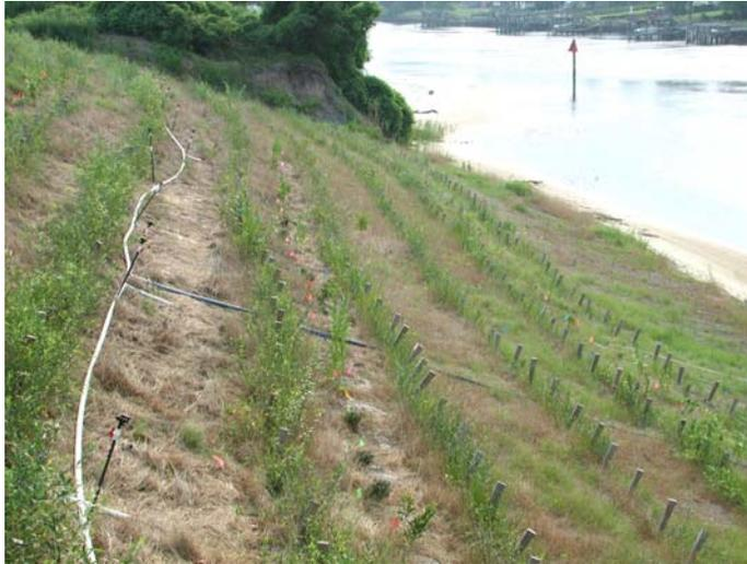
**Figure 2.20: Fascines with erosion control fabric on a slope along the Atlantic Intracoastal Waterway.**
