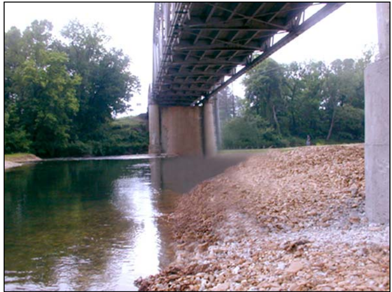
Figure 14. Site 10 on the Barren Fork River below Hwy 51 Bridge
