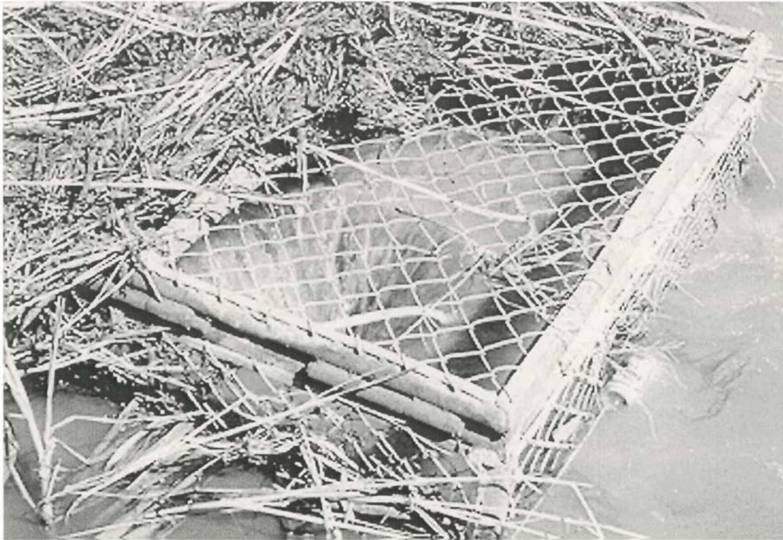
Figure 24. Photograph of the debris screen covering the drop inlet structure of a recharge well.
