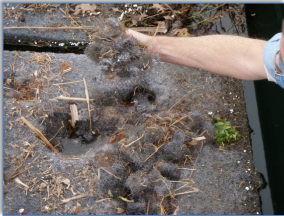
Figure 20 Area assumed to be damage by river otter activity.
