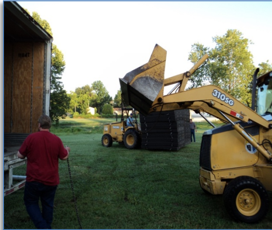
Figure 1 Offloading floating wetland media.
