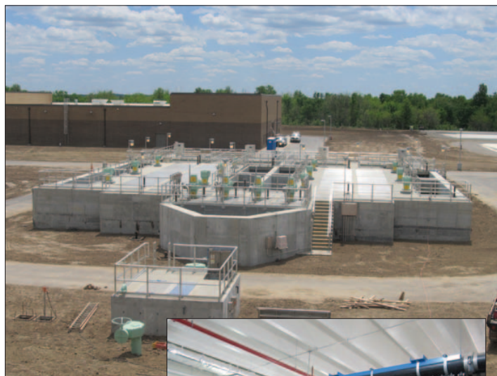
Above: Pretreatment units at Broken Arrow's new Verdigris Water Treatment Plant. The plant is capable of treating up to 20 MGD and can be expanded to treat up to 40 MGD.
