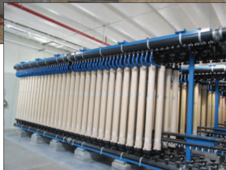
At Right: Advanced membrane filtration system, capable of filtering out extremely small particles and microorganisms, including giardia cysts and cryptosporidium oocysts, to meet new EPA requirements.
