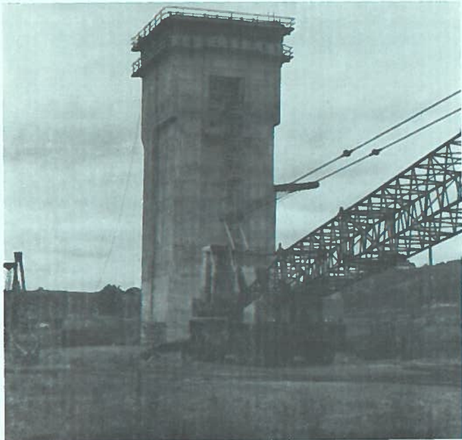
This 130-foot tower houses the control gates at the Arcadia Lake site on the Deep Fork River one and one-half miles southwest of the town of Arcadia and five miles east of Edmond. Construction of the Corps of Engineers project continues on schedule, according to Project Engineer Dennis Frazier, and completion is expected in 1987.
