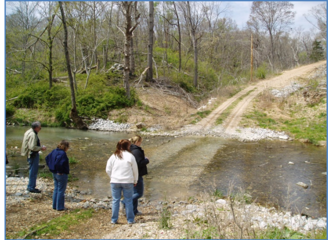
Low water crossing sediment control project at Demonstration Farm in Spavinaw Creek, part of Tulsa’s water supply basin.
