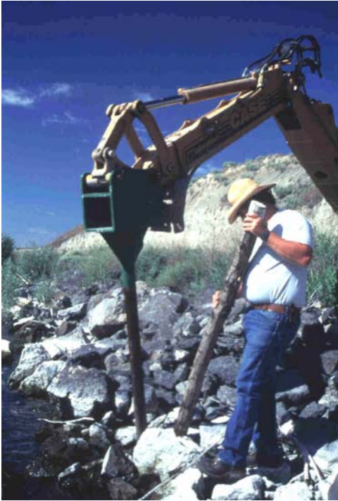
Figure 10. Cottonwood pole being inserted with aid of stinger
