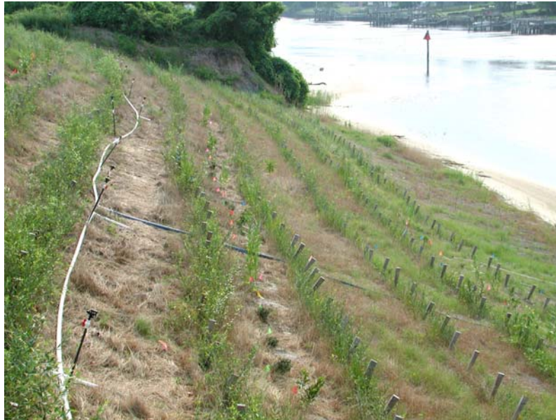
Figure 23. Series of fascines installed on very sandy soil to prevent rills and gullies from overland wash
