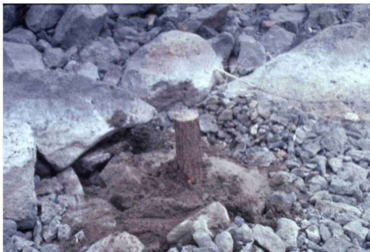
Figure 12. Completed installation of cottonwood pole with stinger
