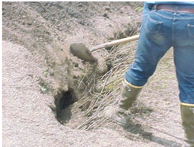
Figure 14. Brush layering; installation of willow cuttings
