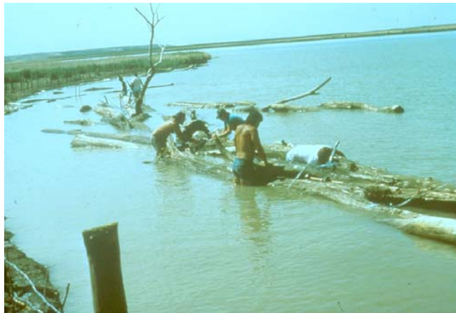
Figure 43. Log breakwater installation, Lake Sharpe, South Dakota, Summer, 1989
