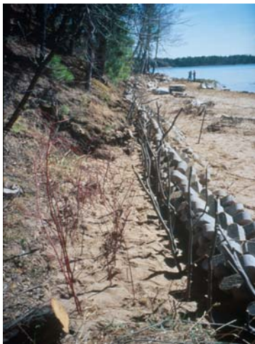
Figure 30. A-jacks immediately after installation
