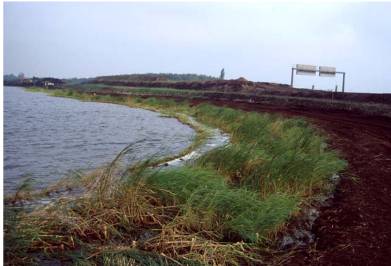
Figure 33. Reservoir in northern Germany with a CGR breakwater and emergent aquatic plants in erosion control mats
