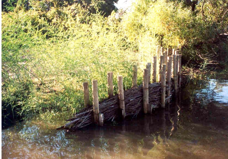
Figure 39. Branchbox breakwater at Lake Wister as viewed from a boat on September 11, 2001
