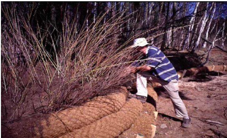
Figure 27. CGRs used to restore bank in figure above.
