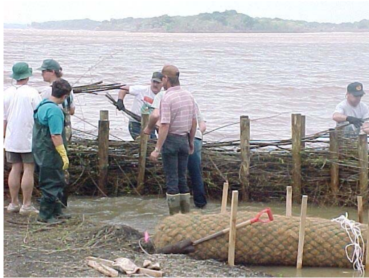
Figure 38. Branchbox breakwater being installed at a workshop/demonstration, Lake Wister, Oklahoma, April 2000
