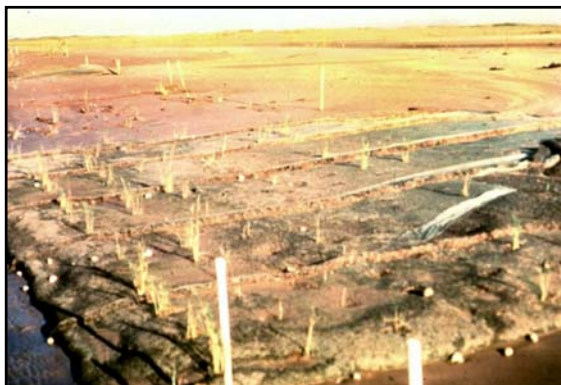
Figure 19. Erosion control mat immediately after installation
