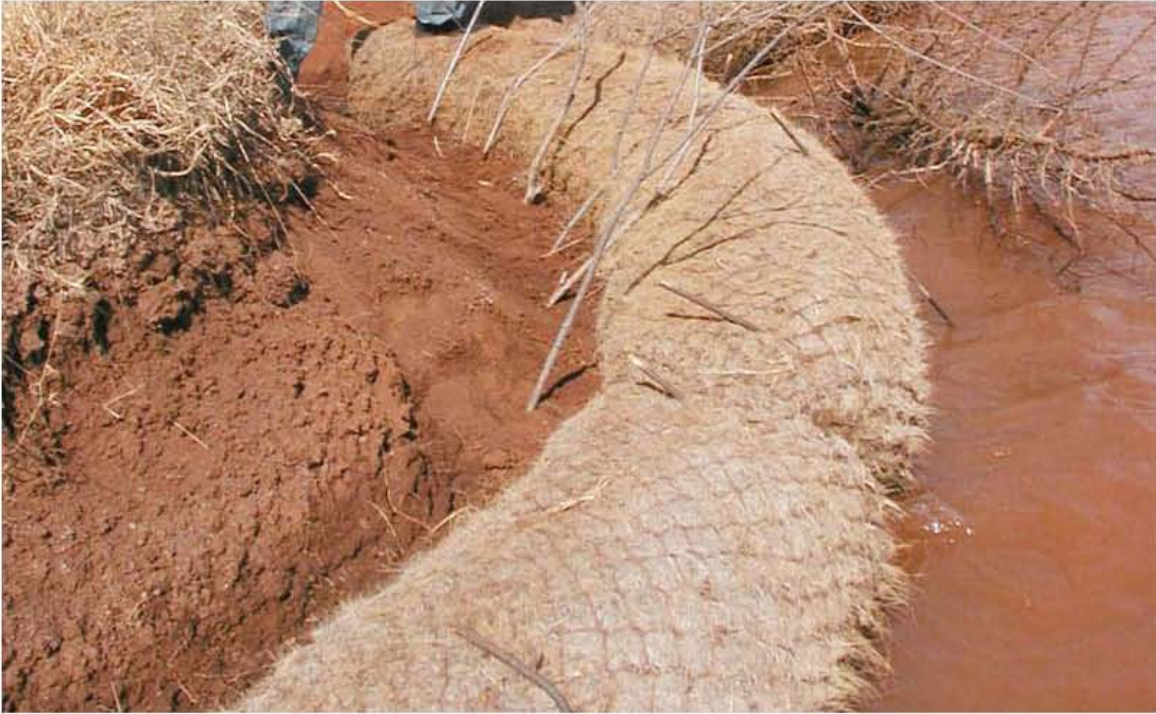
Figure 25: Erosion on escarpment backfilling CGRs
