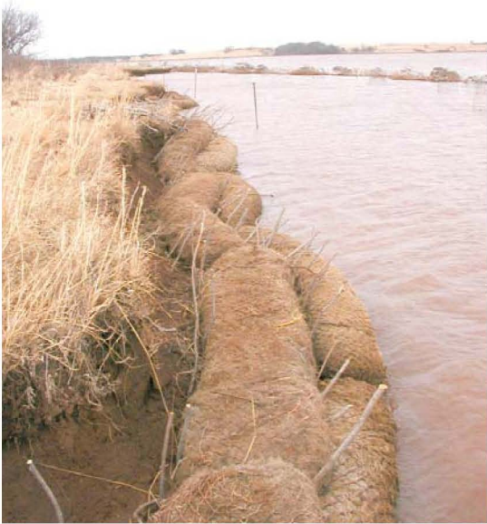
Figure 12: Newly installed CGRs at Site 1 with dormant willow cuttings at 16 inch intervals
