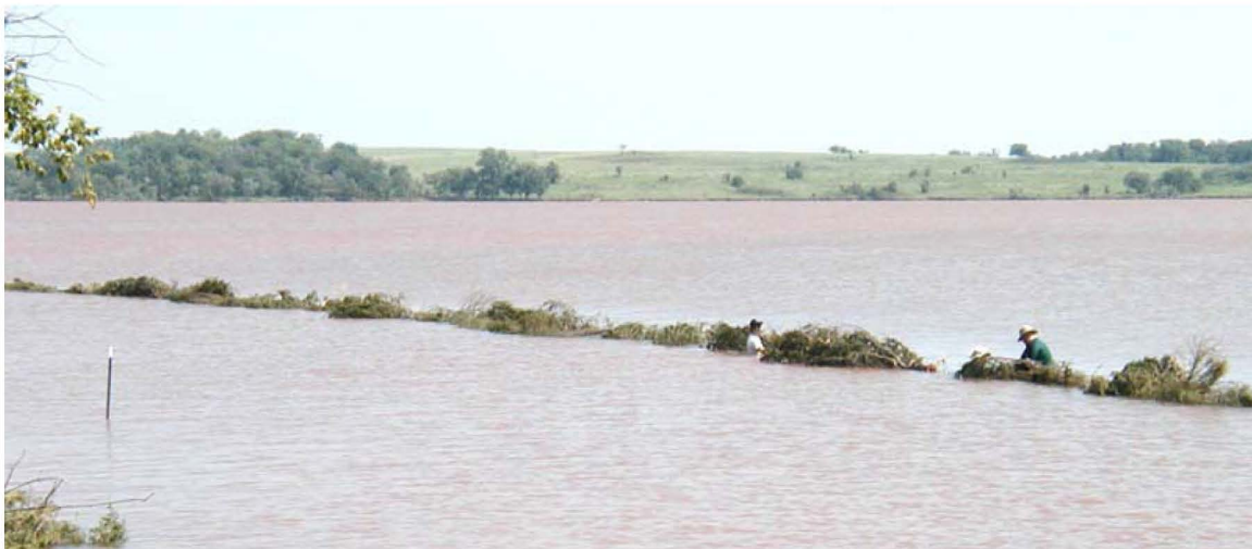
Figure 10: Site 1: Installation of Cedar Tree Breakwater
