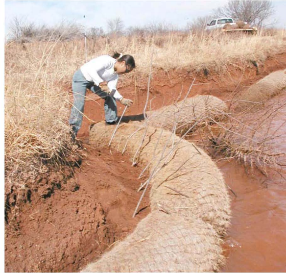
Figure 13: Driving one-foot deep holes for willow cuttings
