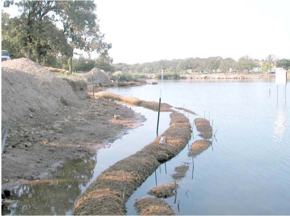
Figure 5: Site 3 CGRs initially installed with rebars, later converted to duckbill anchors.
