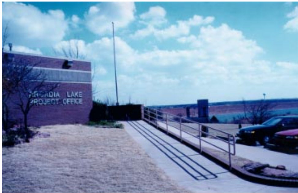
Figure 5.1 Lake Arcadia project office with dam in background
