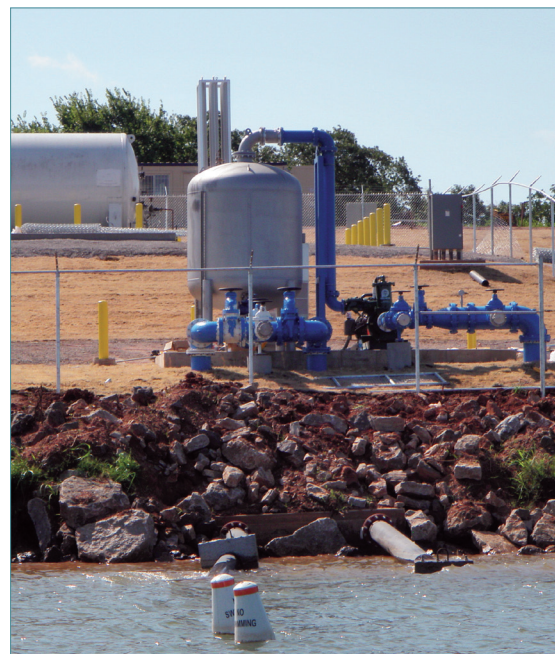
Dissolved oxygen injection system at Lake Thunderbird
