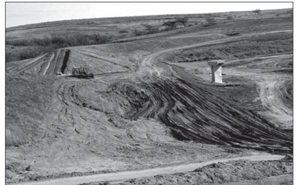
*Reconstruction in April 2000 of a small flood control dam in Roger Mills county, one of 6 dams built in the Sergeant Major Creek Watershed from 1948 to 1963. This site was selected for reconstruction as a result of a hazard classification change due to downstream development, structural problems with the principal spillway, and excessive foundation seepage.*
