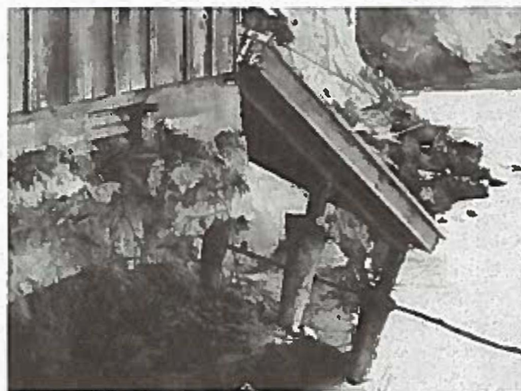
The river under cut the deck, encroached on the foundation and swept away fences, trees and septic tank.
