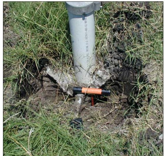
Figure 1. Photograph of water well with an open, unsealed annular space.
