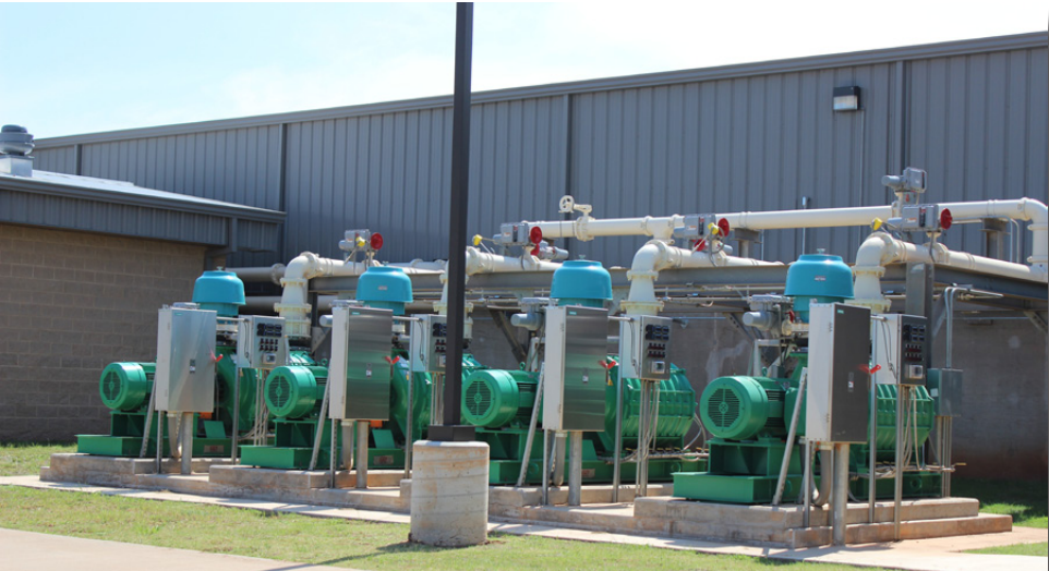
Blowers for the Sequential Batch Reactor (SBR)
